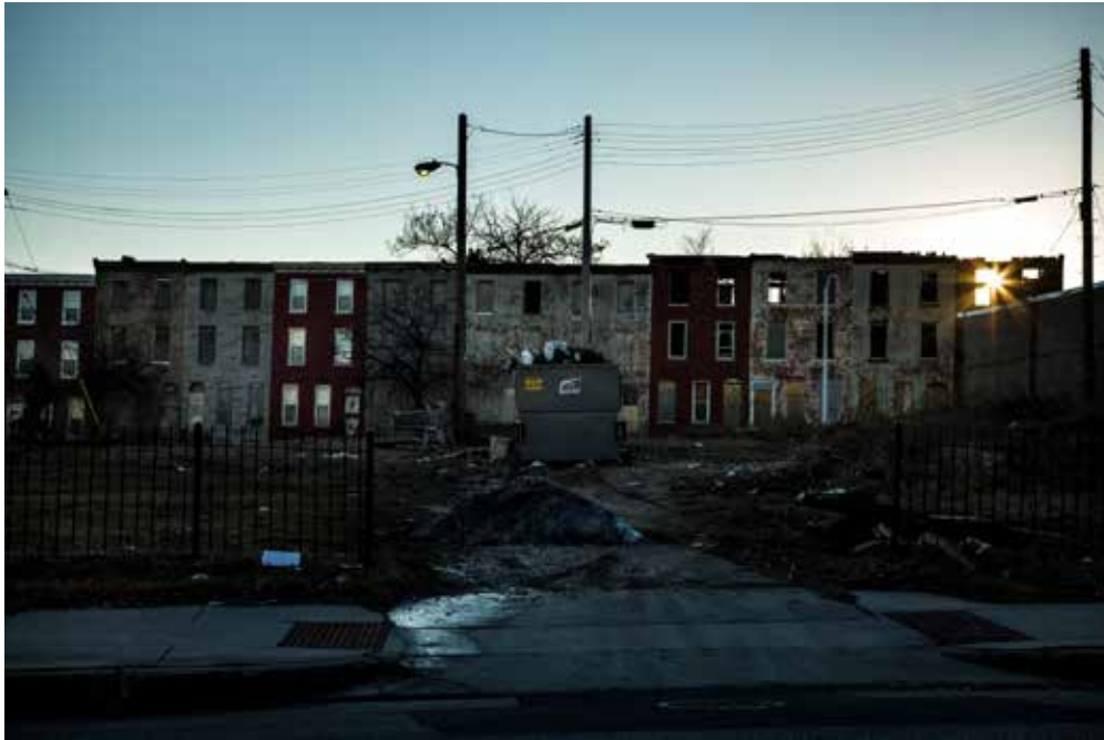
FIGURE 15. Abandoned Homes in Sandtown Baltimore (2016). Photograph by Justin Tsucalas.
